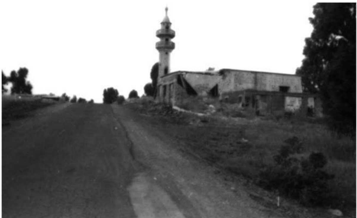
1) The village of Al Khushniyeh before it was destroyed by the Israelis following the 1967 occupation, and the Mosque of Al Khushniyeh abandoned after the 1967 war and
