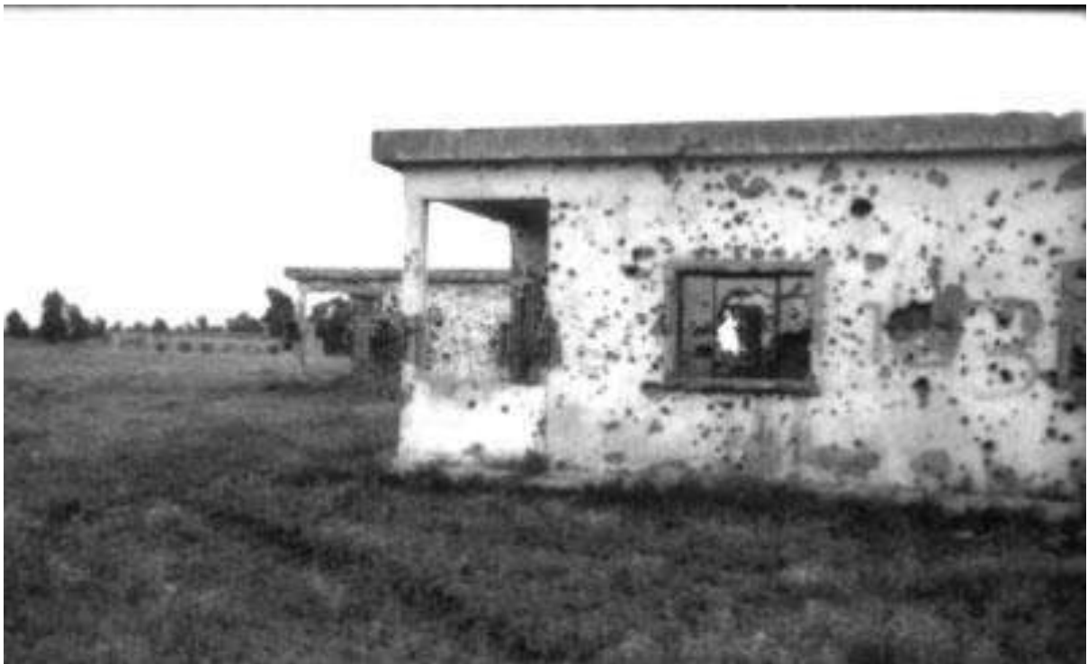
4) Buildings destroyed by military training, Ein-fiet (above) and Al Mansoura (below), Golan.
