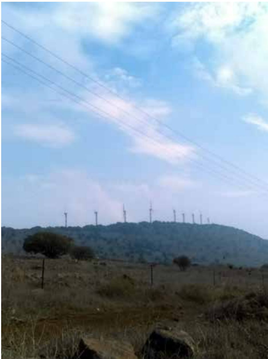
Golan Heights Wind Farm, the only wind farm in the Golan, near Quneitra. These turbines have a hub height of about 30 meters. The Project's turbines have a hub height of 125 meters.
