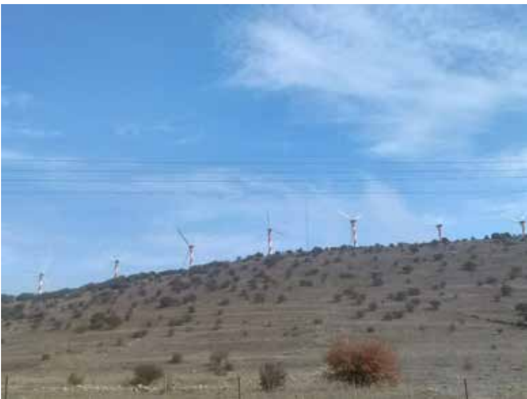
Golan Heights Wind Farm, the only wind farm in the Golan, near Quneitra. These turbines have a hub height of about 30 meters. The Project's turbines have a hub height of 125 meters.
