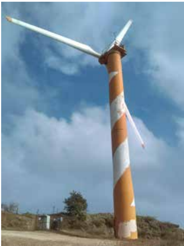
Turbine at Golan Heights Wind Farm, the only wind farm in the Golan, near Quneitra. This turbine has a hub height of about 30 meters. The Project's turbines have a hub height of 125 meters.
