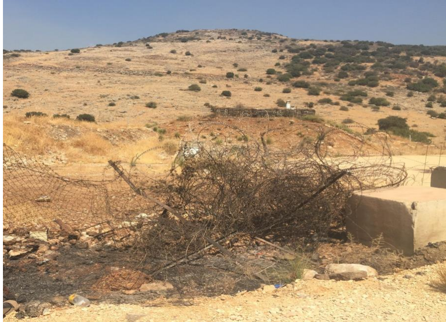
A broken fence surrounding a minefield
